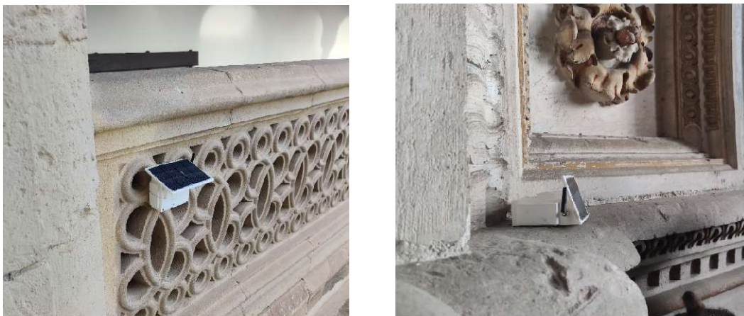
Figure 2: Smart tags installed on the “San Jerónimo Monastery” site (Granada).
