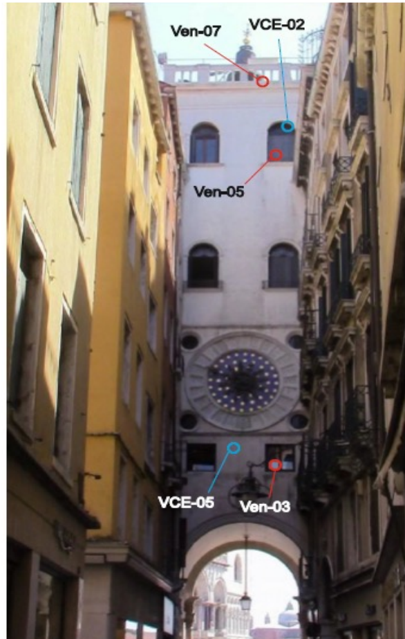
Figure 56: Location of the smart tags (red circles) on the external walls of the Clock Tower, and of the dataloggers (blue circles) inside the building.
