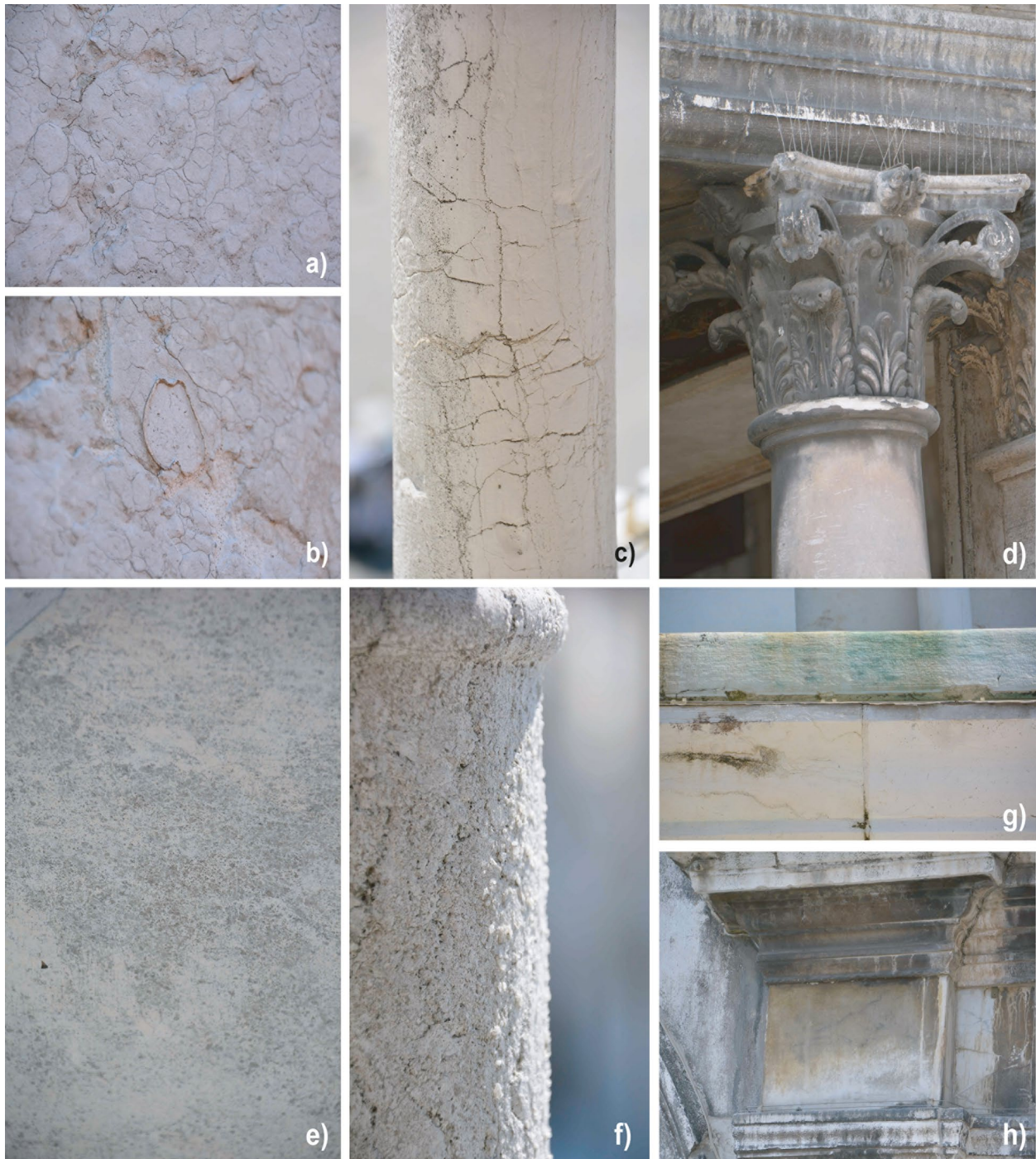
Fig. 6 Features induced by material loss: a, b differential erosion on Ammonitico Rosso from Verona slabs (eastern façade), c microkarst on Istrian Stone small columns (western façade). Discoloration and deposit: d black crusts on Istrian-stone Corinthian capitals (southern façade); e soiling on Scaglia Rossa slabs (western façade); f efflorescence on Istrian Stone small columns (western façade); g greenish staining on Istrian Stone (western façade); h yellowish patinas (southern façade)
