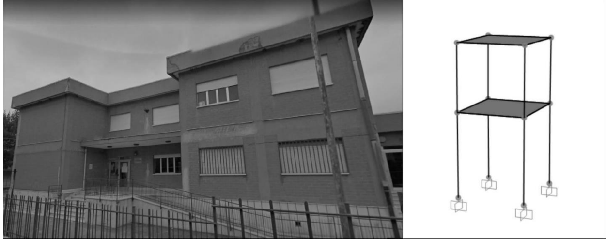
Figure 2 – Concept of 3D reduced-order model by means of a two-story tavolino structure, applied on the B10 case study building (see also Fig. 5).
