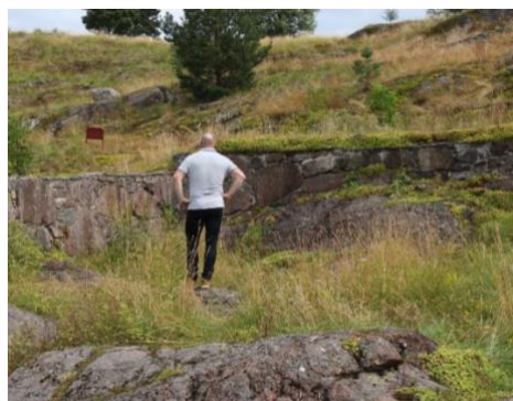
Figure 36 Detail taken inside the ruin
