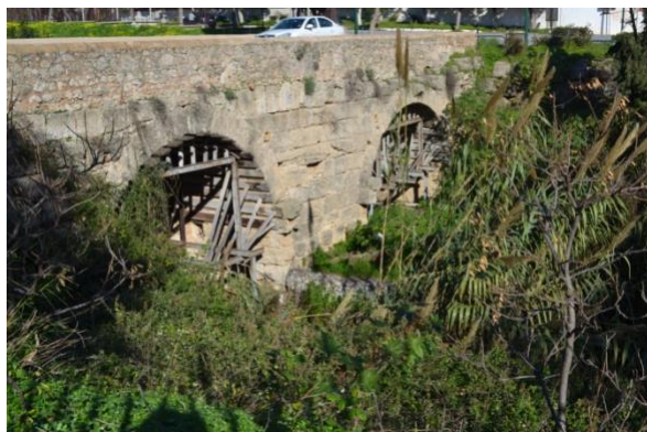
Figure 6 The Roman bridge east facade
