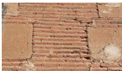
Figure 18 Rammed earth construction, locally named as "tapial".
